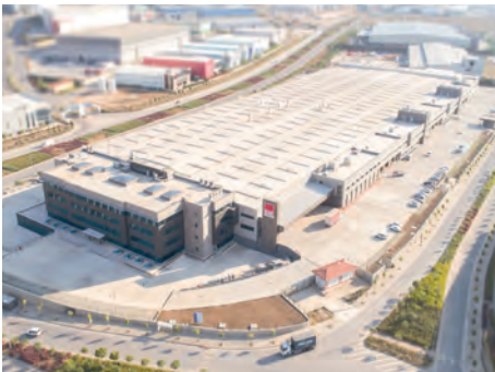
Plant 4 Busbar Factory Kocaeli / TURKEY
