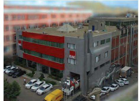
Plant 3 Technology Factory Istanbul / TURKEY
