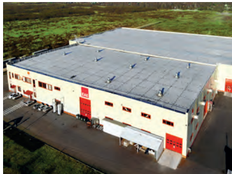
Plant 5 Busbar & Lighting Factory Aleksandrov / RUSSIA
