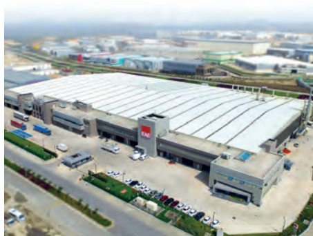
Plant 2 Cable Tray Factory Kocaeli / TURKEY
